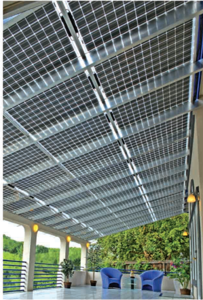
Patio Awning: Solar Living Design Lakewood, CO
